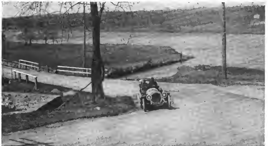
This Turn, In the Vicinity of Kensico, Is Particularly Difficult.
